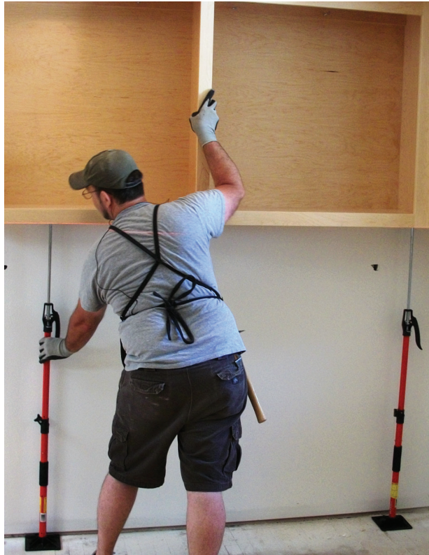
B Designed to support upper cabinets when the base cabinets are not yet in place
